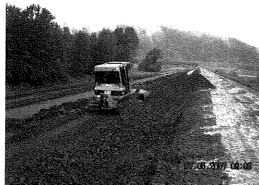
50+00 PLACING BASE MATERIAL
